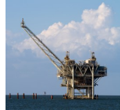
Offshore Rig Maintenance
