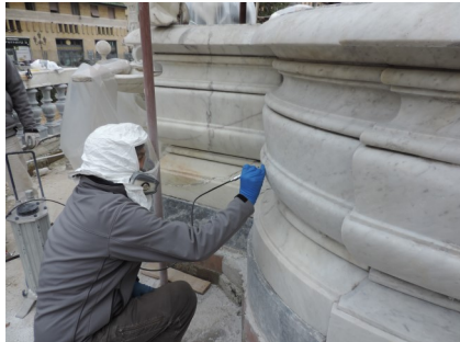
Cleaning the famous Trevi Fountain in Rome 2015 with an Ibox9 Blaster and Pen Gun.
